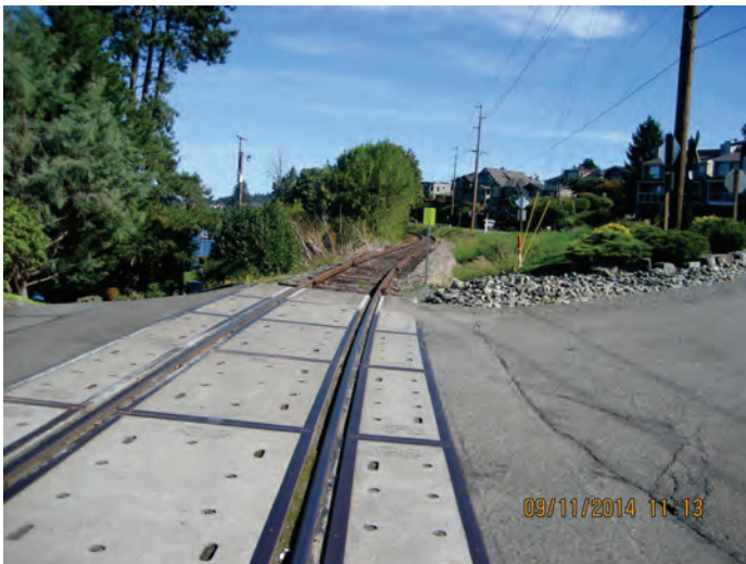
Milepost 5.3 looking north near the intersection of North 33rd Street and Mountain View Avenue North (September 11, 2014)
