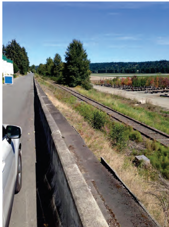
Redmond Spur Milepost 3.0 looking north near the intersection of Willows Road SE and 141st Avenue NE (September 11, 2014)
