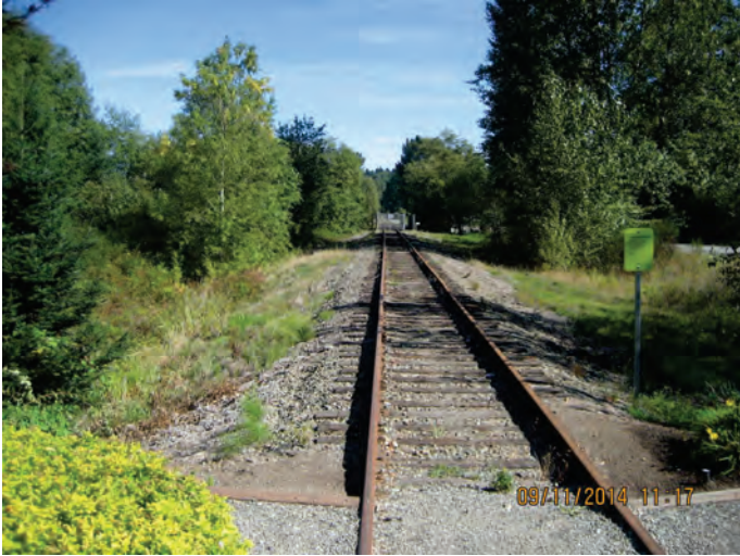
Milepost 6.1 looking northeast near the intersection of Wells Avenue North and Lake Washington Boulevard North (September 11, 2014)
