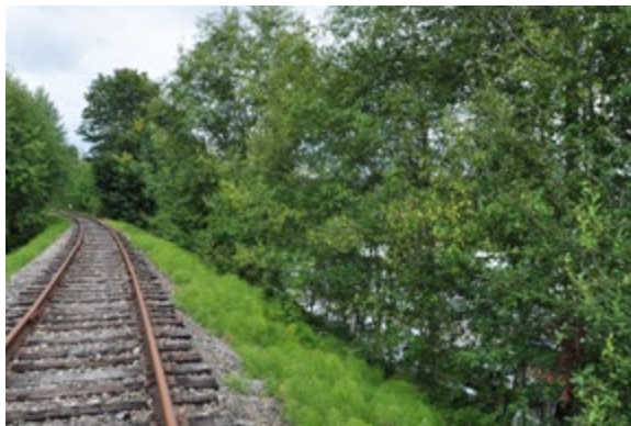
Steep embankments, as seen to the right in this photo, are common within the ERC right-of-way.
