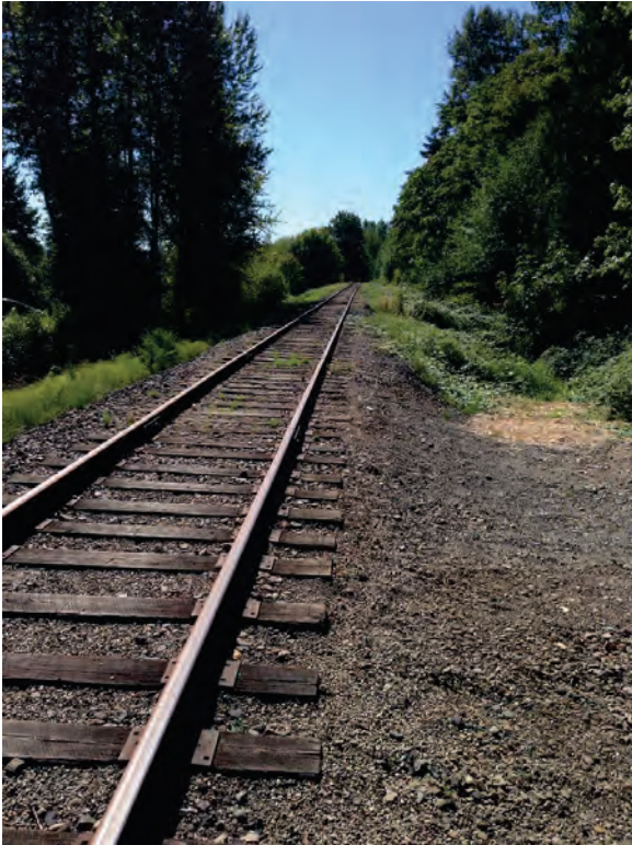
Milepost 21.0 looking north near the 139th Avenue NE crossing (September 11, 2014)
